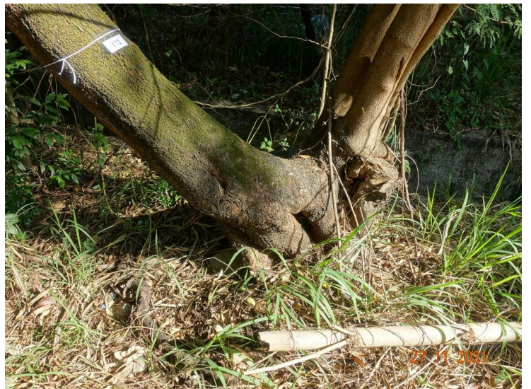
T72 LOWER TRUNK AND GROUND CONDITION - FELL
