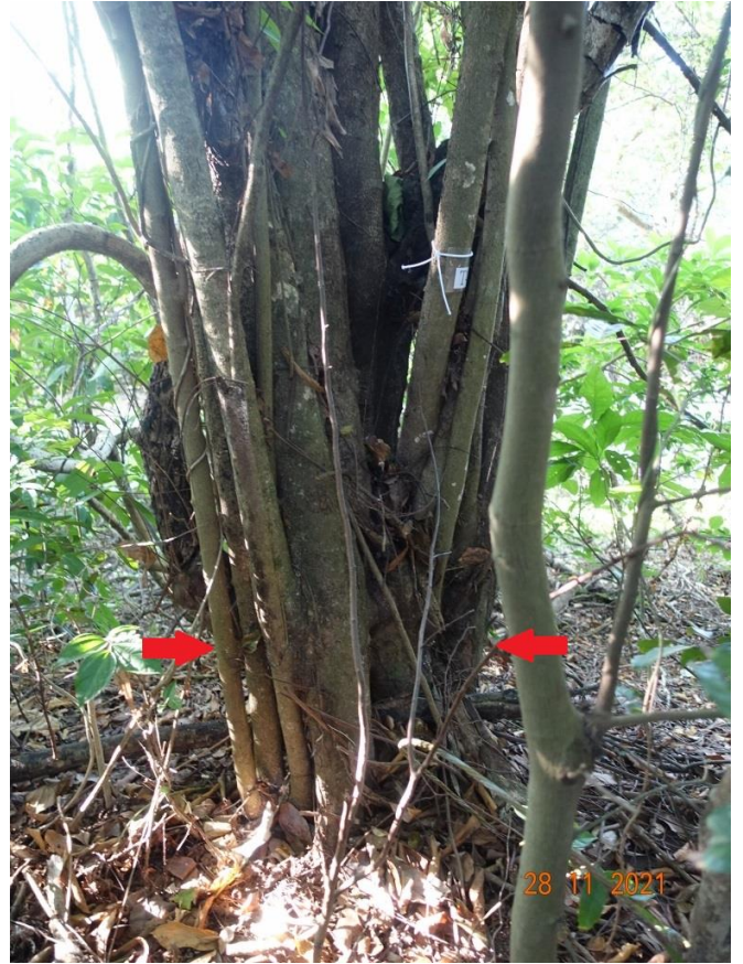
T45 LOWER TRUNK AND GROUND CONDITION - FELL
