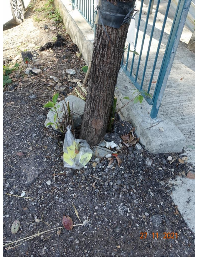
T61 LOWER TRUNK AND GROUND CONDITION - FELL
