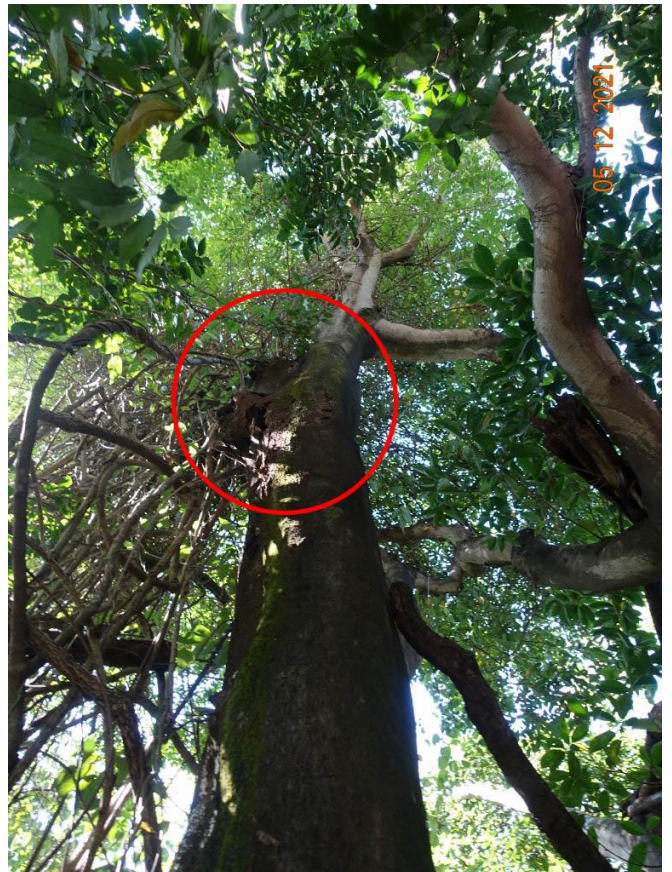
T150 DEFECT - DECAY ON MAIN BRANCH- FELL
